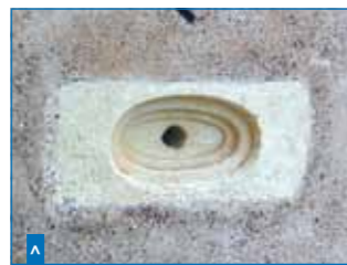
Orifice de surveillance
